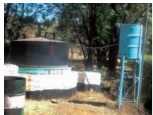
Gas collection tank resting on the concrete-built digester. Pipes / tubes at the top of the gas tank supply the house with methane gas, Botswana. (Reuben Sebeg)
