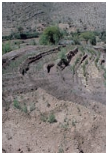
Photo 1: Main canal for diverting flood water from seasonal rivers to the field. Lateral embankments are stabilised with stones.
