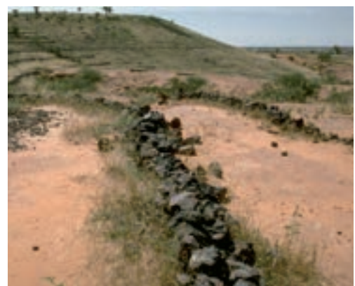
Top: Konso Terraces in Ethiopia. (Rima Mekdaschi Studer) Top middle: Fanya juu terrace with napier grass, Kenya. (Hanspeter Liniger) Bottom middle: Vegetative strips along contour line for reducing surface runoff and erosion, Kenya. (Christoph Studer) Bottom: Stone lines catching run-off water and fertile soil sediments, Niger. (Hanspeter Liniger)
